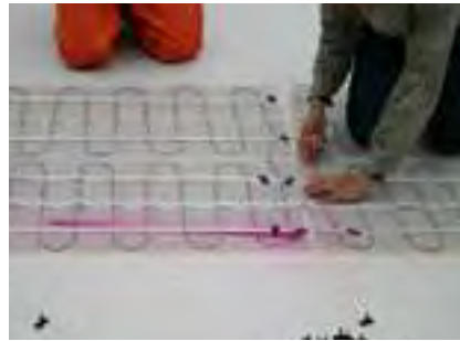
DSVF-90 (DEVIheat™ 90S) mat is laid out.
