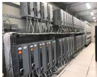
iSave 70 energy recovery devices, APP 86 pumps, VLT® AQUA Drives, and DST P40I pressure transmitters in the Sarlux SWRO plant
