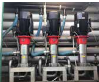
iSave 70 energy recovery devices, APP 86 pumps, VLT® AQUA Drives, and DST P40I pressure transmitters in the Sarlux SWRO plant
