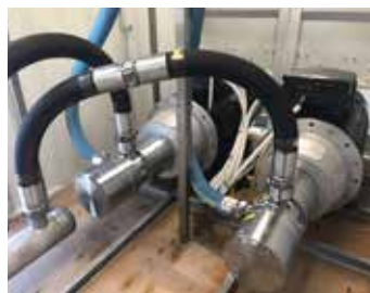
iSave 70 energy recovery devices, APP 86 pumps, VLT® AQUA Drives, and DST P40I pressure transmitters in the Sarlux SWRO plant
